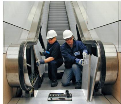
The escalator modernization is protected with barriers to minimize any safety risk for passengers. KONE keeps the customer and end-users informed about the progress of the project and the installation phases. KONE also takes care of the safe, environmental recycling or disposal of the old equipment. After handover, we can ensure that your modernized escalator continues to operate reliably in the future, with regular, preventive KONE Care™ maintenance.
